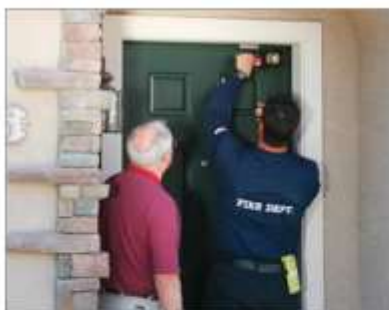
1. The Columbus Fire Department installs the Knox Box
